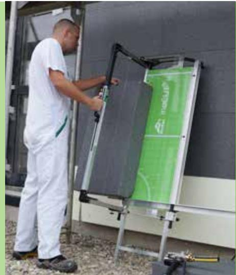
The **inoCUT ic3** revolutionises thermal cutting of ETICS rigid foam panels on the construction site.
