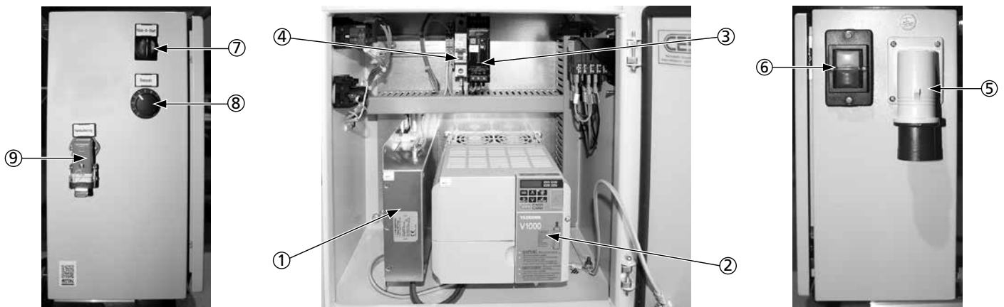
View of the switching cabinet from the left-hand side
