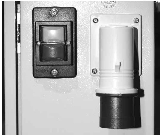
3-pole 230 V / 16 A feed supply CEE plug (right) on the switching cabinet
