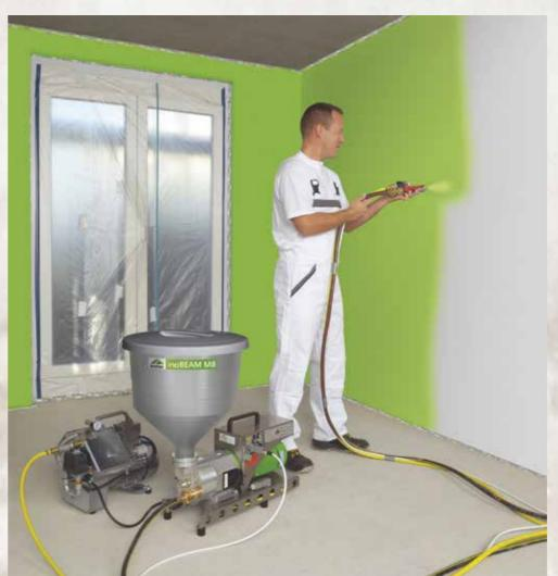
The InoBEAM M8 delivery pump can be used universally: From decorative fine layers, liquid woodchips and paste-like structural plasters to mechanically applying paste-like ETICS adhesives.
